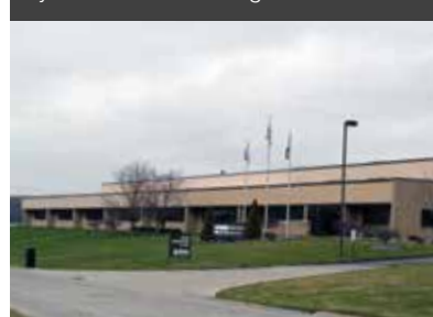
Wadsworth, OH - Industrial Profile Systems manufacturing.
