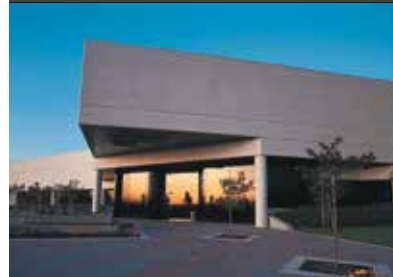
Rohnert Park, CA - Electronics Business Unit and Headquarters for Electromechanical NA.
