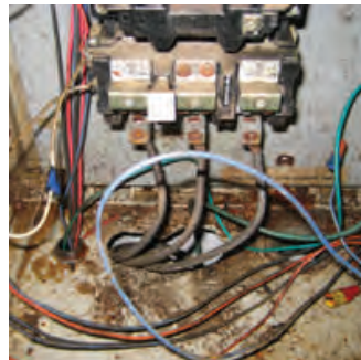
Corrosion leads to premature component failure
