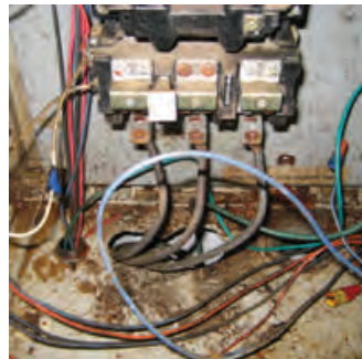
Corrosion leads to premature component failure
