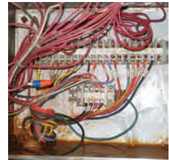
Water accumulation in electrical cabinet
