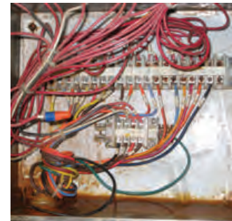
Water accumulation in electrical cabinet
